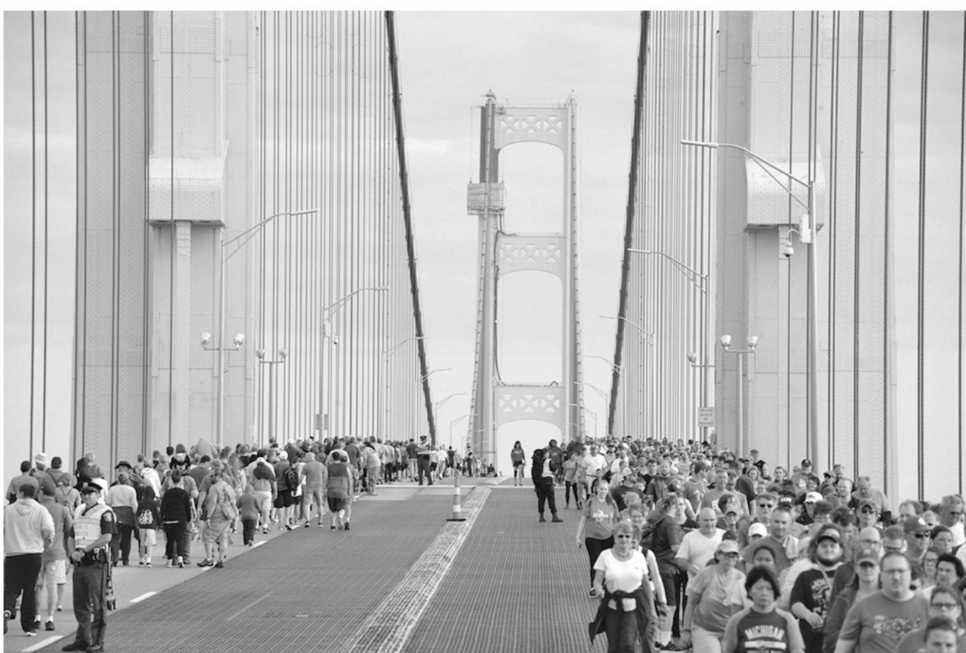
The 2018 Annual Bridge Walk included a first ever occurrence: walkers going both north and south on the bridge at the same time. © 2018 MDOT PHOTOGRAPHY UNIT
